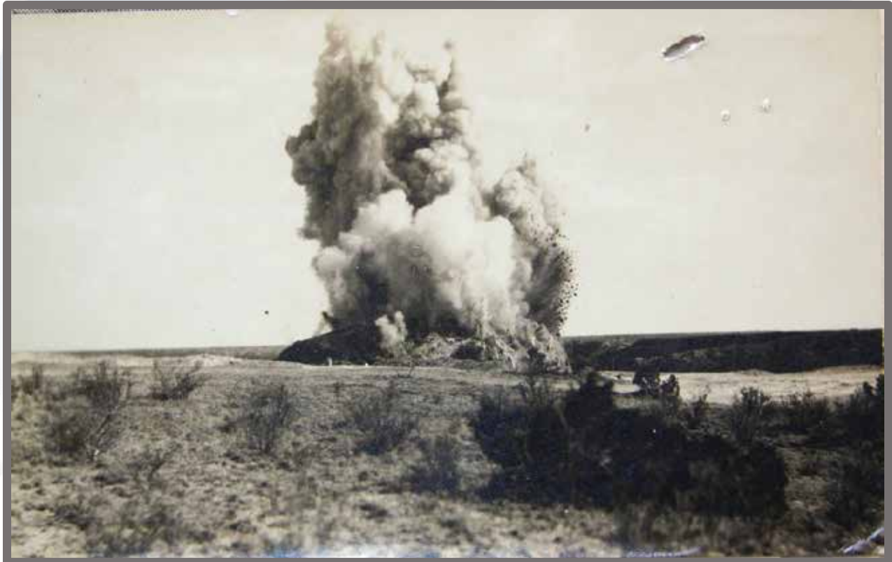
Real Photo Postcard of a Blast: “Shot in caliche pit Apr. 9, 1934” “Note rise in ground and how stones stayed in air to be photographed.” Signed EAK (E.A. Kingsley, NPS superintendent overseeing construction.) (Images from: NARA. Denver, CO.) Photo and caption provided by Lisa Jackson.
